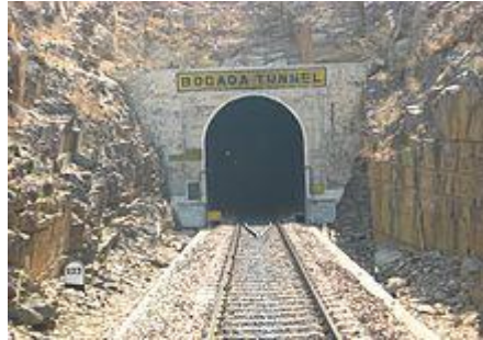
Railway Tunnel in Nallamala
